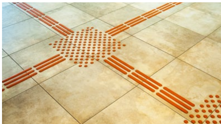
At the town hall a tactile guidance system leads people to their destination. (Photo: Verbandsgemeinde Nieder-Olm)
