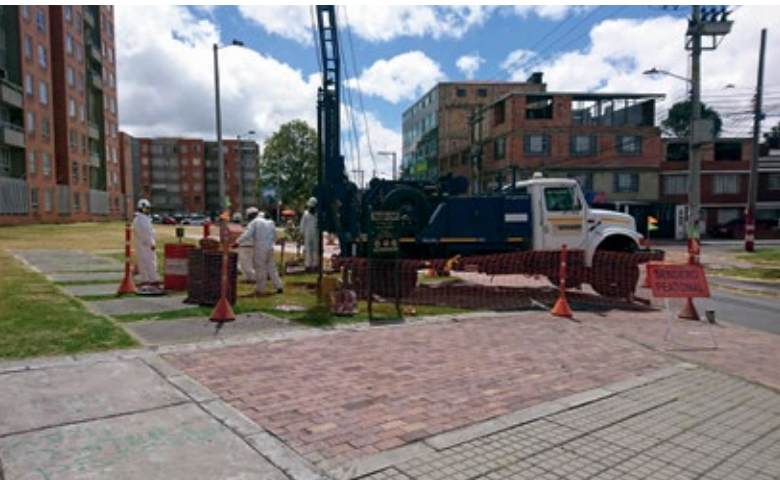
The project team from Stuttgart and Bogotá drilling for samples. Before new buildings are erected in the Colombian capital, the site has to be examined for contamination from previous usage. © Hermann J. Kirchholtes
