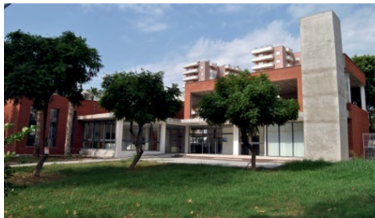
A very neat and tidy building site – the 'Mezitli Active Aging Center'. This was painstakingly planned and implemented together with the Tempelhof-Schöneberg District. The second storey was added on the initiative of the Turkish partners. © Okan Saydam, Mezitli
