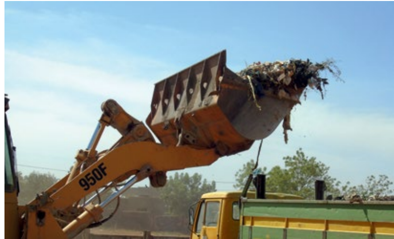
To better manage the masses of waste in Kati a wheel loader was purchased through the partnership project with Erfurt. © Georg Ohlmann
